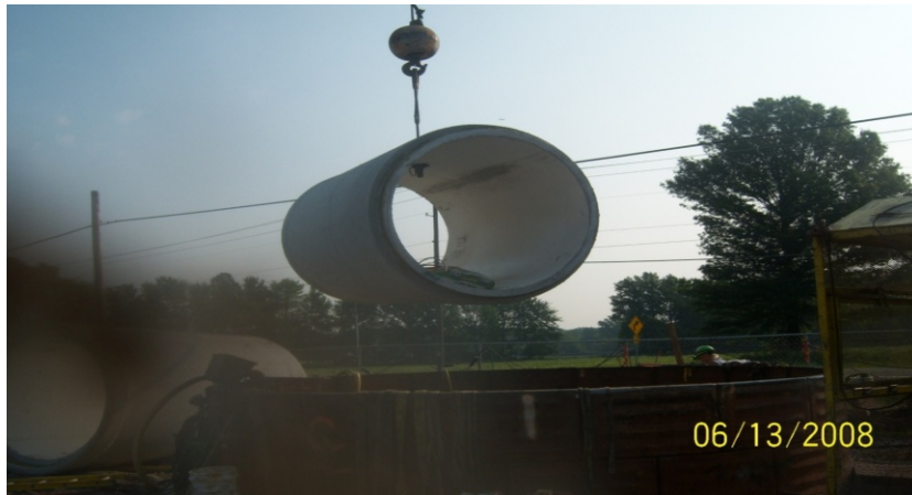
Reinforced Concrete Pipe (RCP) T-Lock Liner
