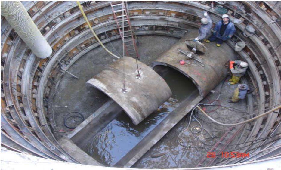
Outfall Shaft – Tied into Existing 84-inch Sanitary Sewer
