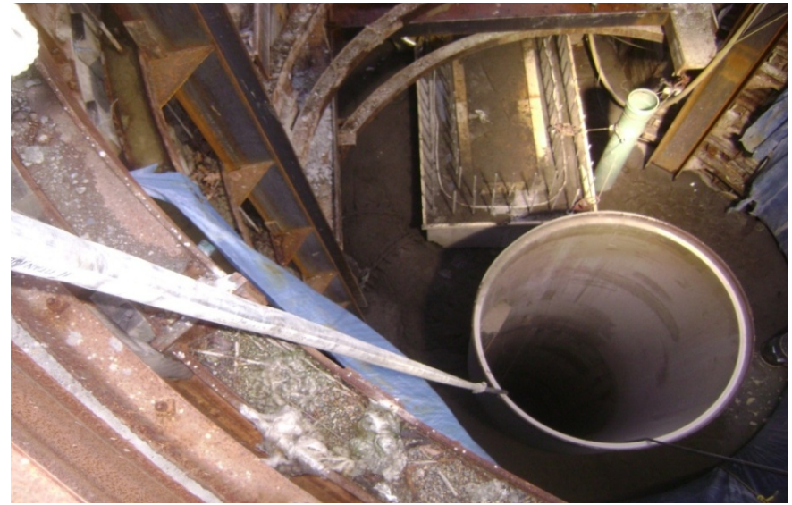
Shaft 4 Tangential Inlet – Tied into Existing 36-inch Sanitary Sewer
